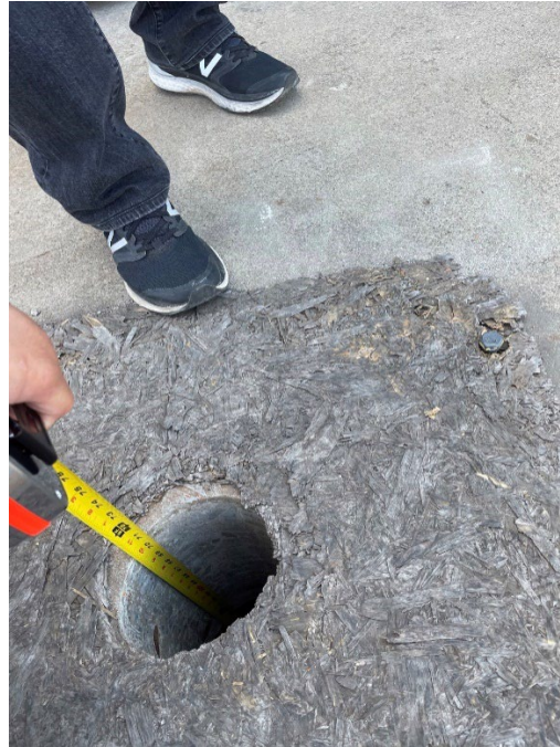
Figure 8: Measurement showing six feet distance between the top sediment layer and top of concrete surface, Wharf, Alameda
