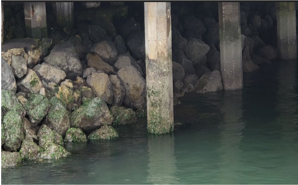
Figure 4: Rip-rap on the Rock Dike, Howard Terminal
